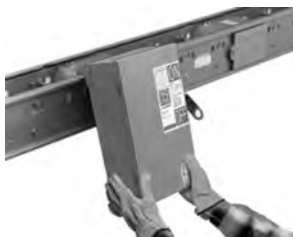
Figure 111 - Plug-In Device Mounting
